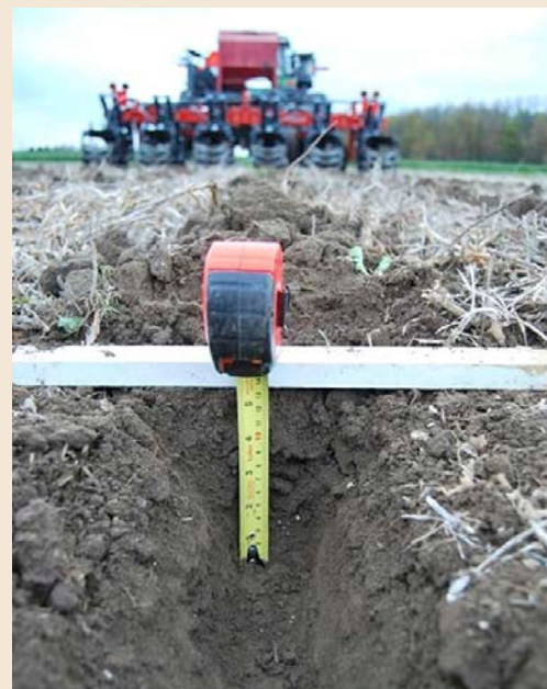
Figure 6. Strip-till fertilizer band placed 10 cm (4 ins.) below soil surface.
